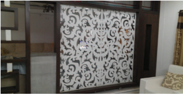
Fig. 5. Mdf jali partition finished with duco paint used by author for residential interiors at Hyderabad, India.
