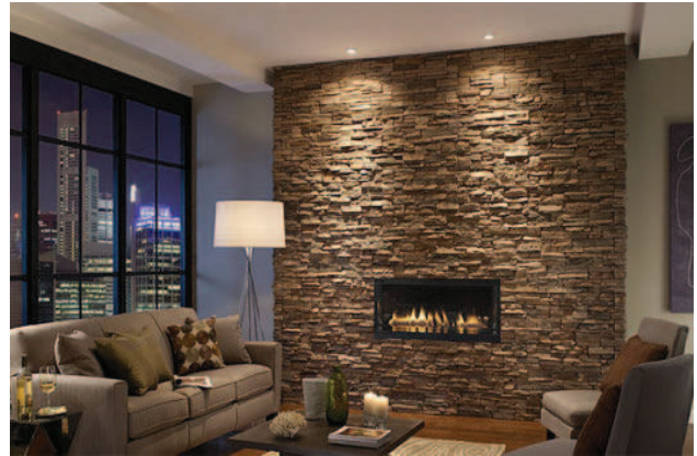
Fig. 6. Cladding: Stone wall as an imitation in interiors
