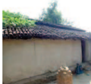
Figure 37. View from Courtyard
