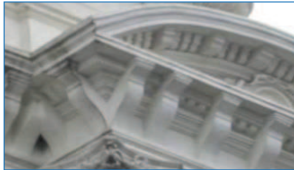
Fig. Workmanship of skilled labors.
